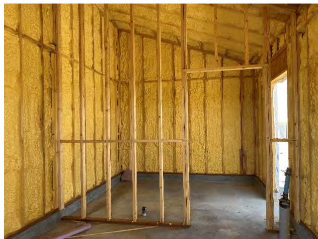
2 – Interior framing/insulation for the chlorination building
