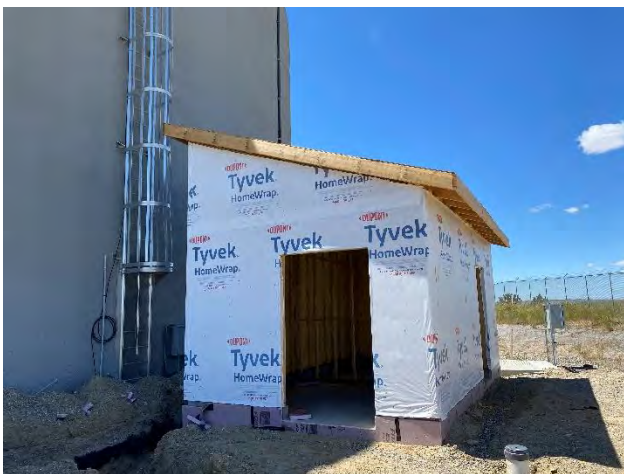
1 – Chlorination building at the Ox Bow reservoir site.
